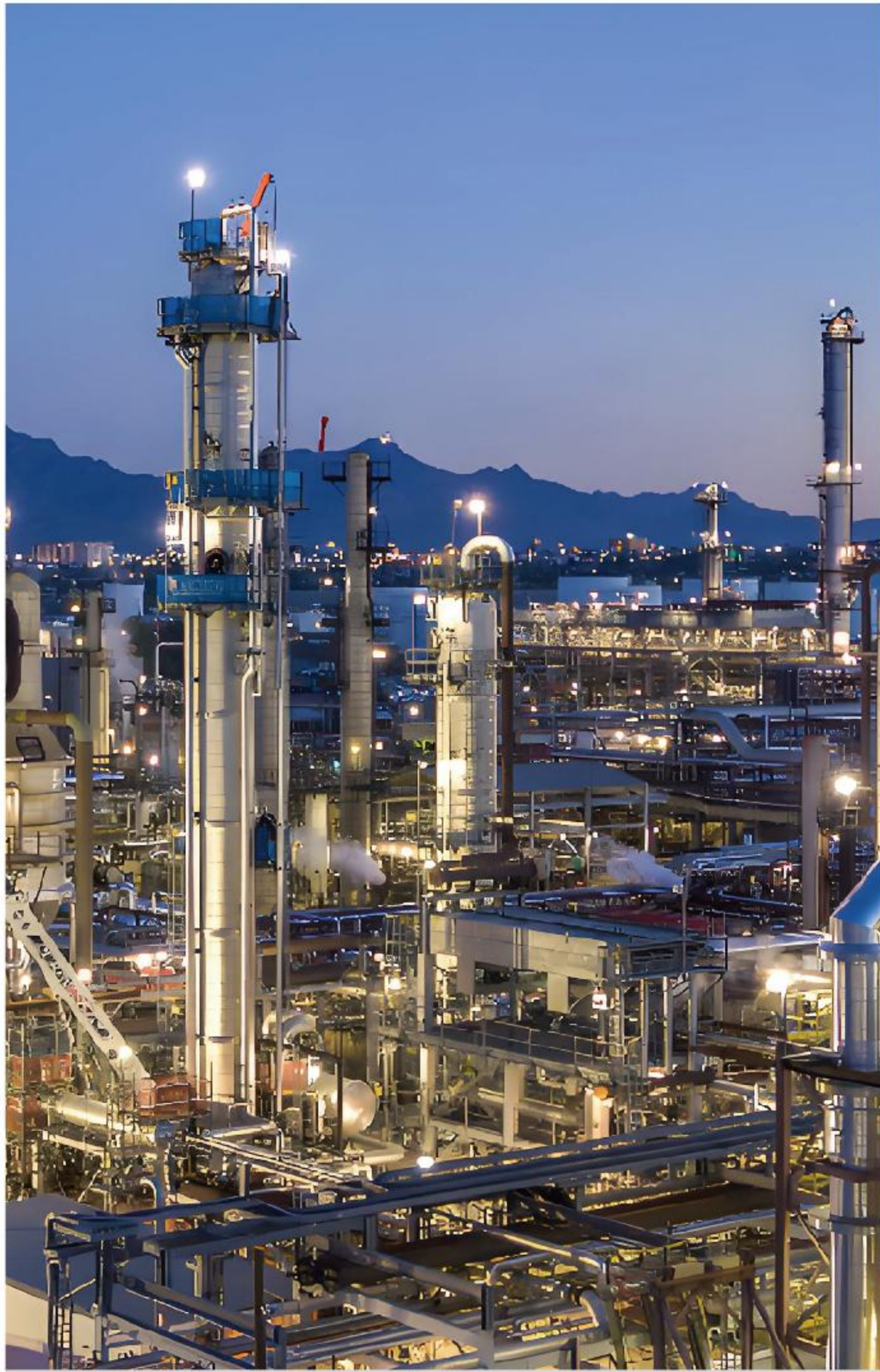
Petroleum and Petrochemical
